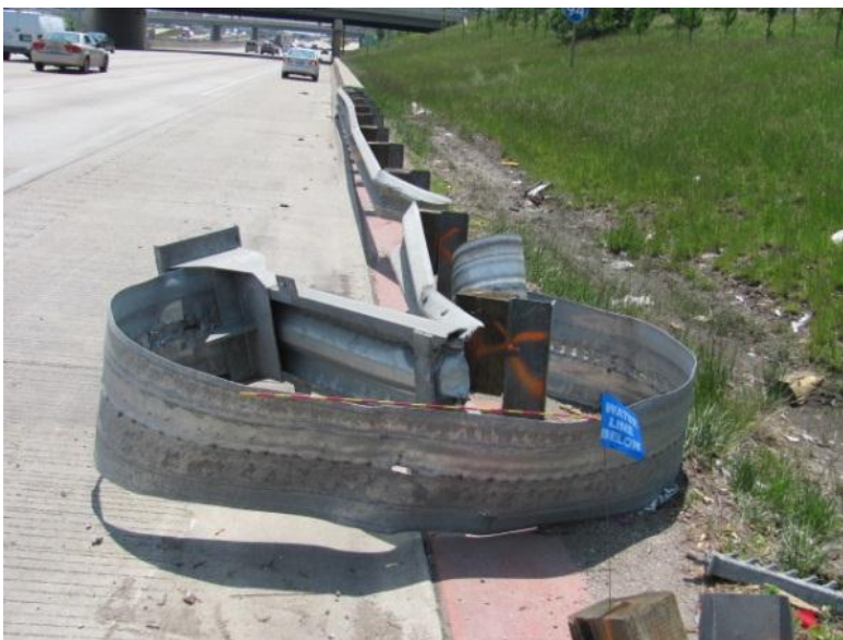
Photo 17 – Post-impact rail condition
