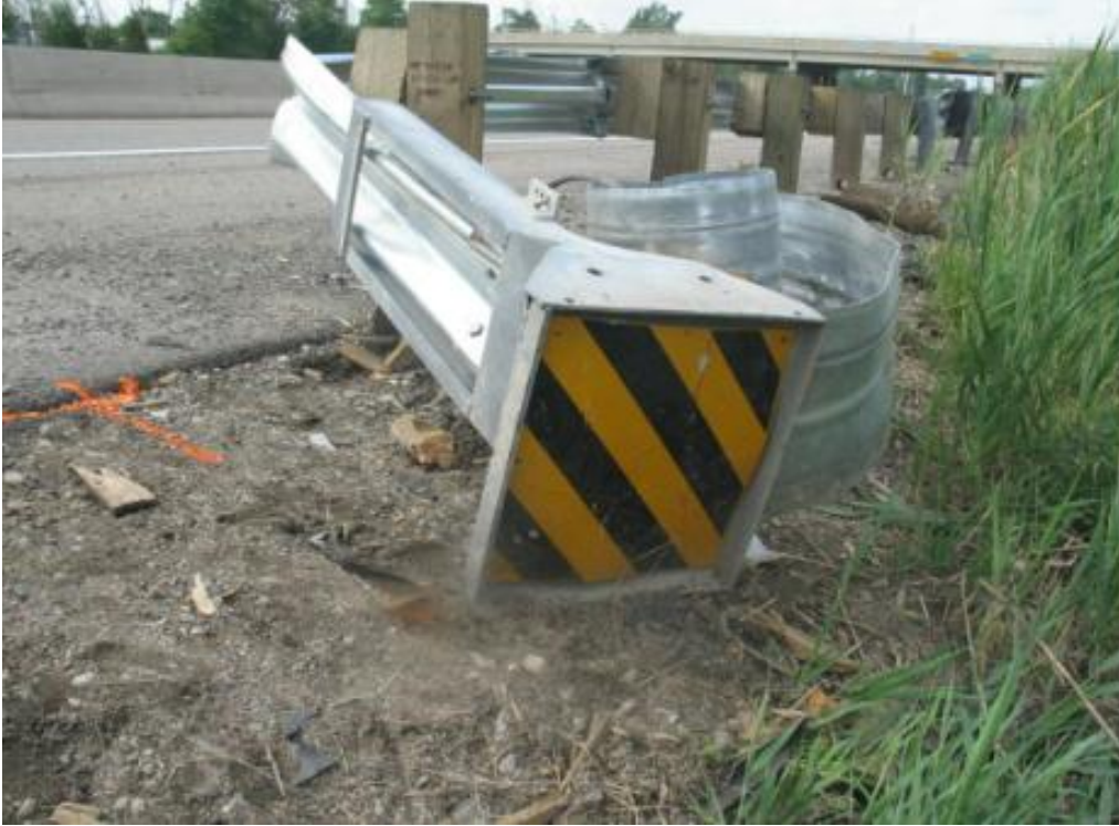
Photo 2 – Close-up of end terminal
