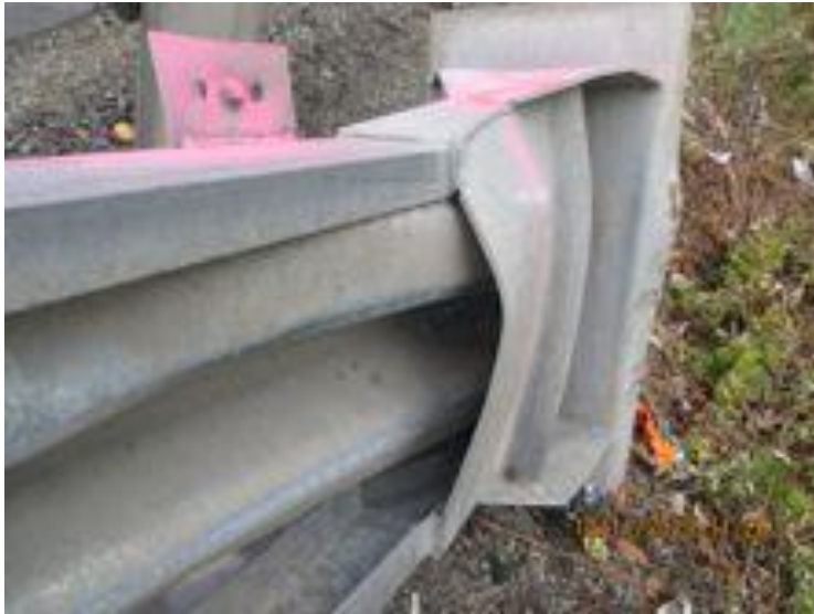
Photo 34- Bowing of reducer sides
