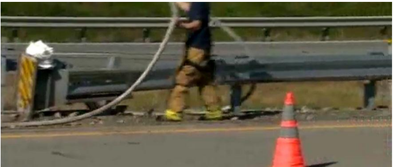
Photo 12 - On-scene photo of terminal after impact
