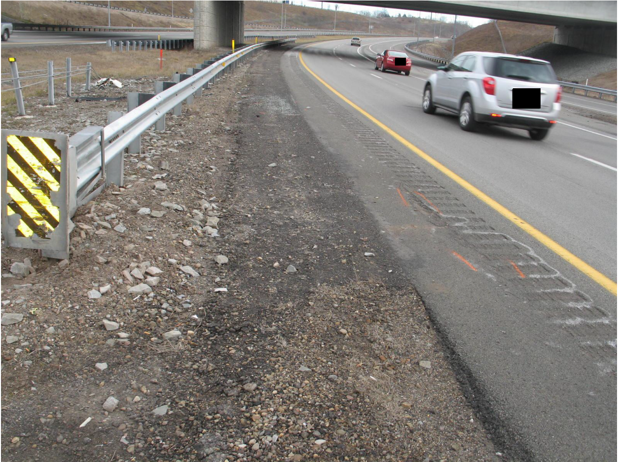
Photo 11 - Repaired terminal at crash site
